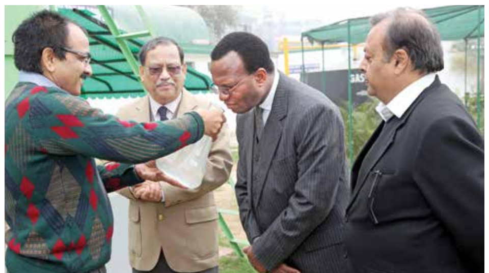
A Sulabh official showing the treated water to His Excellency Mr. Alexandre Cécé Loua which has been taken out from the Sulabh Effluent Treatment Plant.
