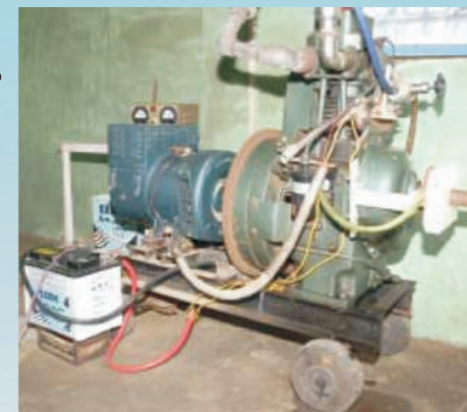
Biogas generator - Operation on gas alone with spark ignition.
