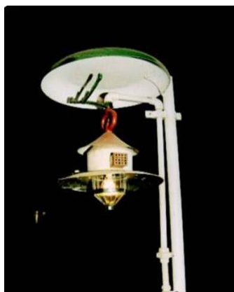
Biogas used for lighting of mantle lamps with spark ignition
